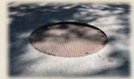
UTILITY BOXES- Typically installed by a utility company but often sink or lift
